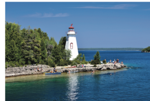
Automated in the 1960s, the Big Tub Lighthouse today is maintained by dedicated community volunteers. This charming site, accessible by road, is popular with swimmers, divers & picnickers.
